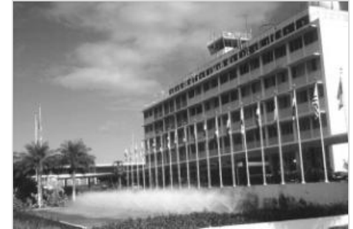
Original structure of the SJU International Airport in San Juan, Puerto Rico.
